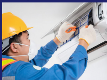
AC Repair & Maintenance
